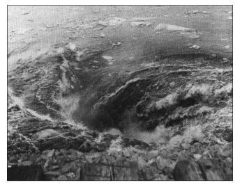
A whirlpool was created by the Susquehanna River flowing through a hole in the roof of a coalmine at Port Griffith, Pa., 50 years ago. To seal the breach, more than 50 railroad cars and 500 mine cars were dumped into it, as were bales of hay, railroad ties, dirt, and rock. It took two days to begin to stop the flow of the water through the hole, which was estimated to be up to 150 feet wide.
